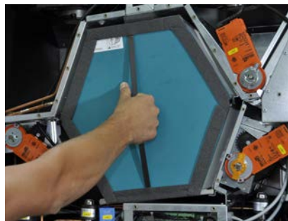
Figure: Counterflow heat exchanger
